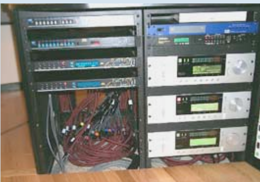
Transparent cabled all digital paths in the new studio with hundreds of feet of Reference AES/EBU Digital Cable.
